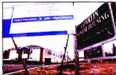
The Conklin Senior Housing apartment complex is located on Conklin Road in the town.
